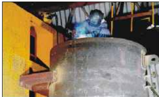
Down Hand welding
