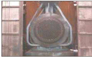
Shot blasting and painting
