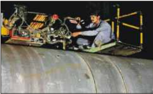
Submerged arc welding
