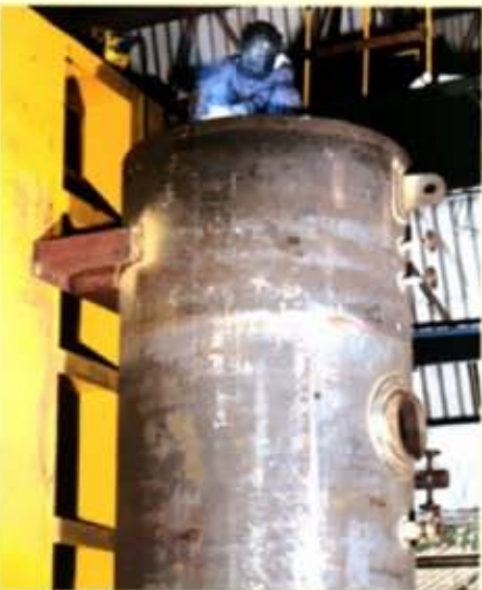
Down Hand Welding
