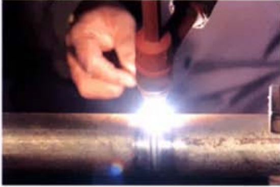
TIG Welding of tubes
